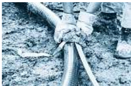
1. Fix the CALPEX®-pipe to one end of the rail, using the tensioning belt.
