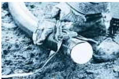
2. Fix the CALPEX®-pipe to the other end of the rail.
